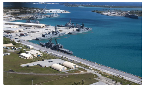
Fleet Piers at Guam
